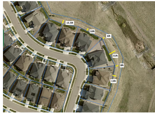
Image: Satellite view of retaining wall, distance from fence to edge of upper wall
