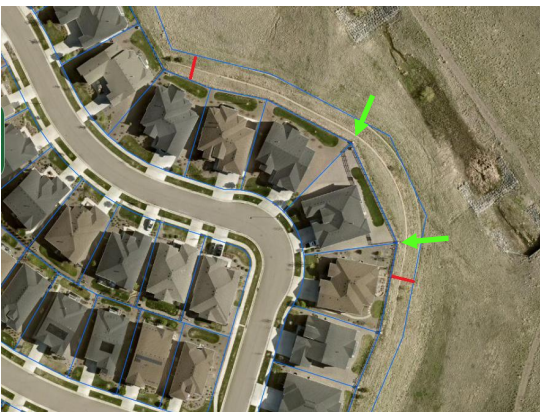
Image: Satellite view of retaining wall, red lines indicate where walls exceed 4ft high
